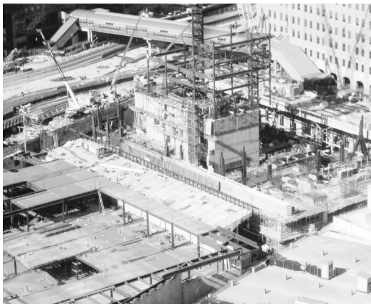
View from above of Freedom Tower (top corner) steel rising.
