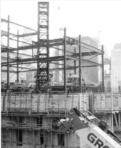
Steel rises on Freedom Tower.
